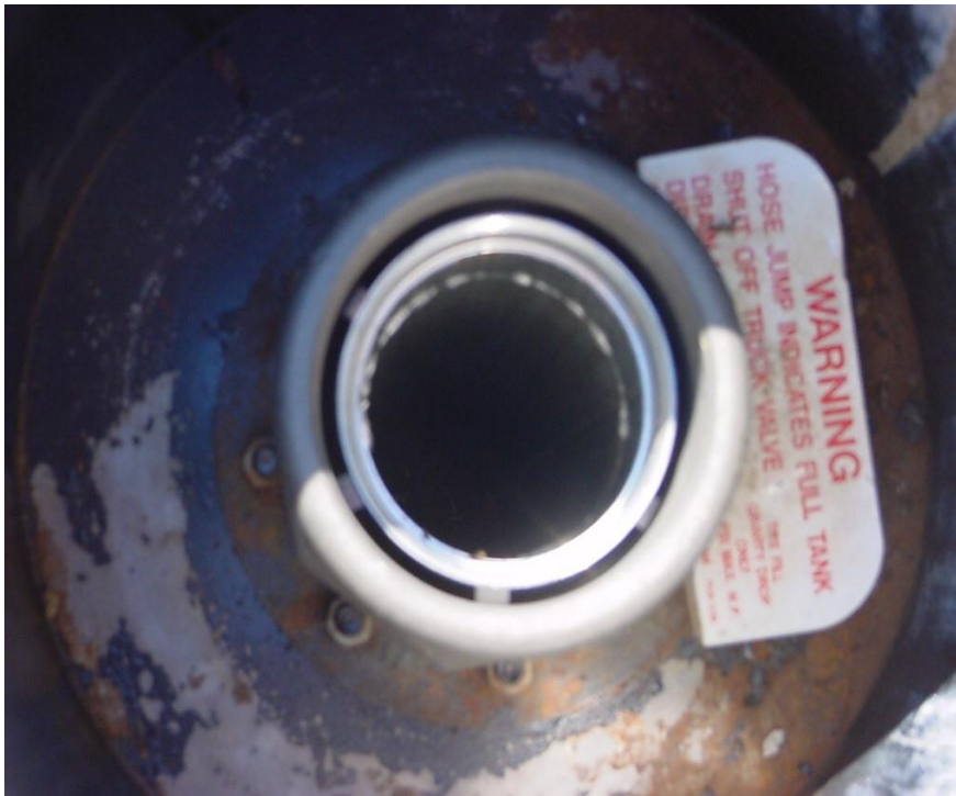
Coaxial Vapor Recovery
