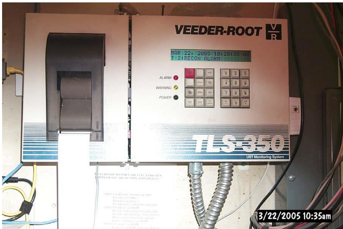
Example of an ATG monitor.
