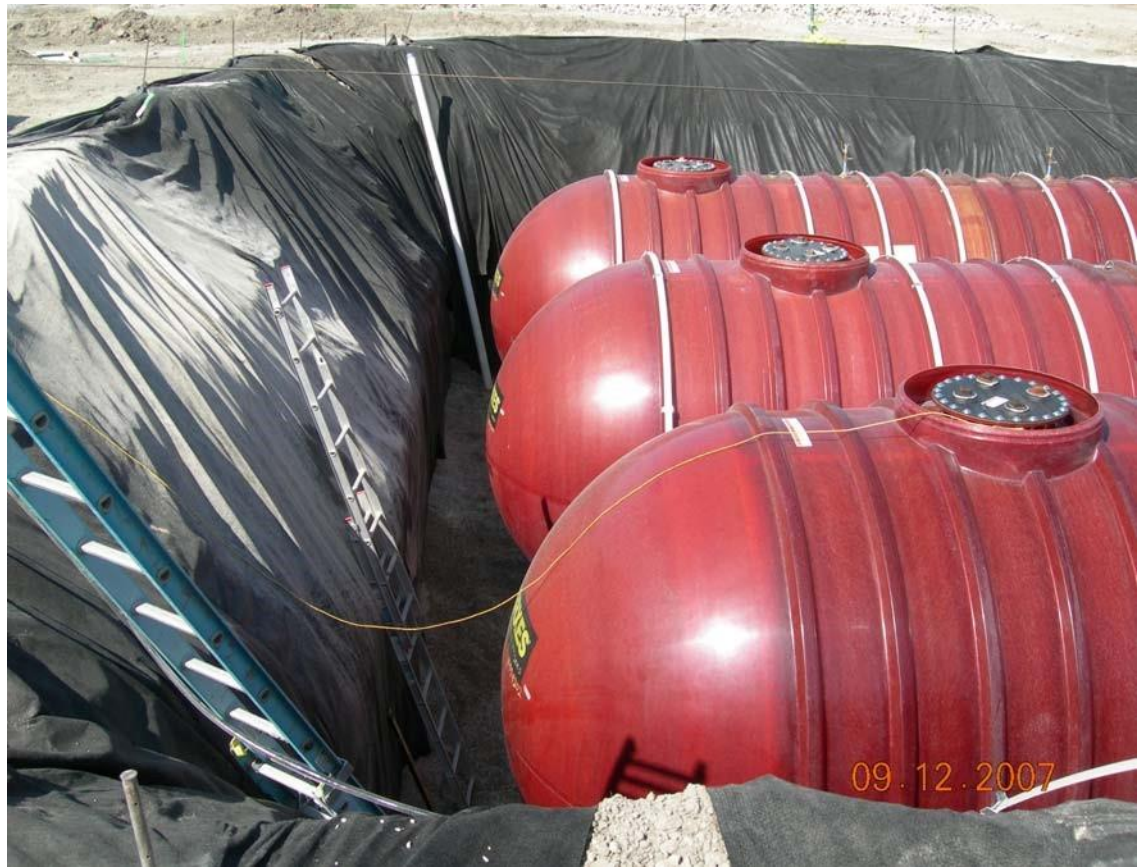
Fiberglass Tanks
