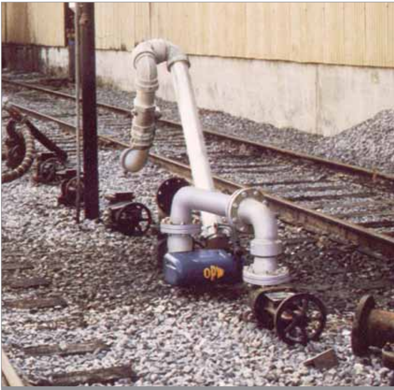
Swivel joints are an integral part of OPW's complete line of loading arm assemblies. This arm replaced hose in a railcar unloading operation.
