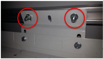
**STEP 12.** Place the mounting foot to the inside of the end panel and mark drilling points. Use a spacer when mounting on uneven surface as shown below. Use a 1" hole saw if the van is equipped with floor mats. Use a 1/4" drill bit for pilot and 3/8" drill for 1/4-20 blind fasteners. Install 1/4-20 blind fasteners on the floor. Refer to blind fastener instruction on page 5. **Always be sure to make sure you won't be damaging wiring, gas lines, or other critical vehicle systems when drilling**.
